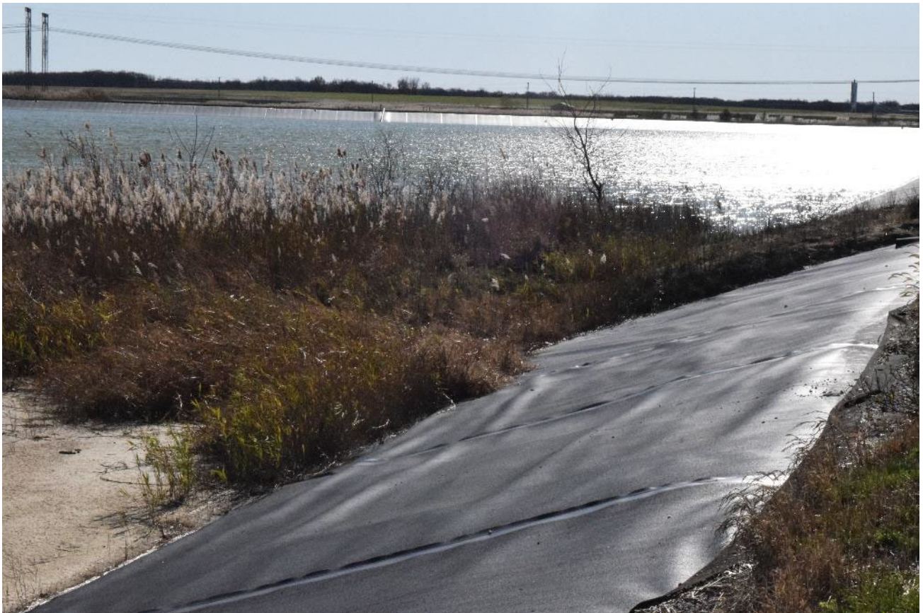
West side – remove small woody vegetation growing on liner at north end
