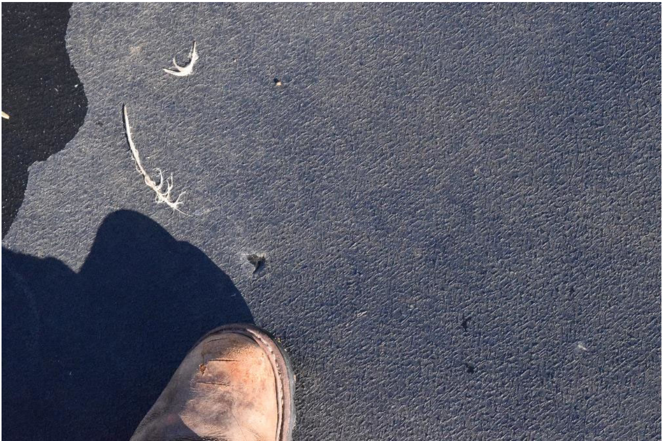
Punctures in liner at inlet – repair
