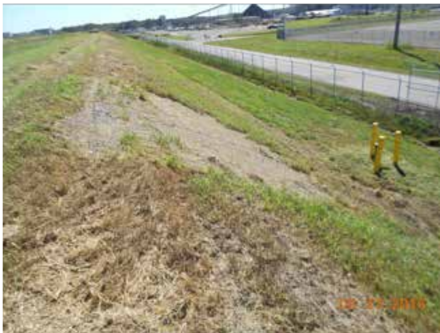
Figure G.4. Photo of 2015 sloughing area after repairs.
